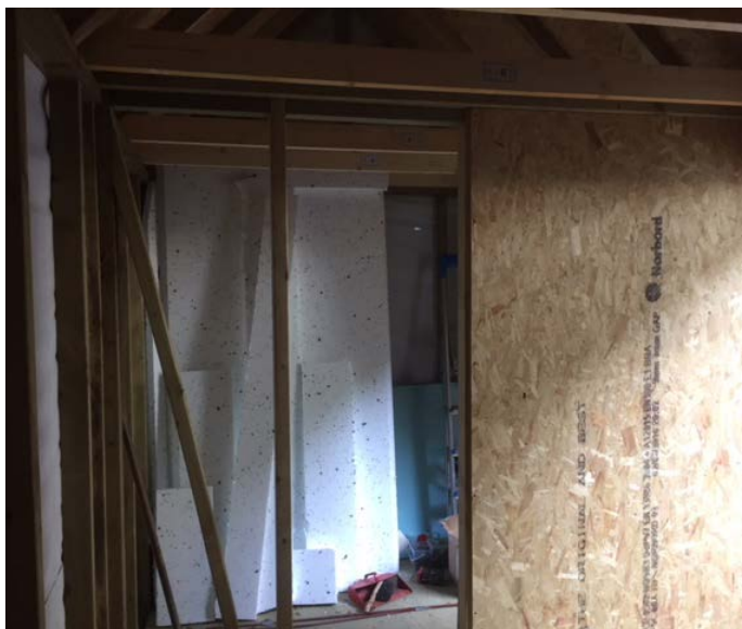
The interior partition wall between drying room and tackle store, with insulation panels. Photo: Doug Harris
