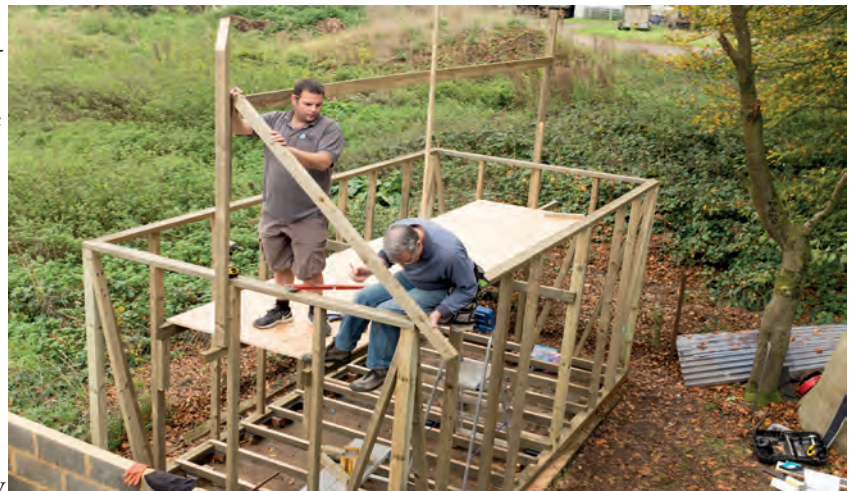
From the lofty heights of the temporary mezzanine-deck, Russ - in serious builder mode (pencil behind both ears), and Brian measure the gable-ends so the roofing can begin. The ridge is on temporary supports.
