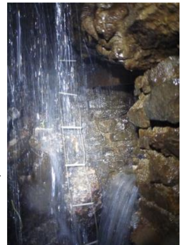
Photo 9. Water entering dug passage from the end of the old adit, 6 th Nov 2013 [Photo: Alison Moody]
