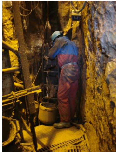
Dave Turner working on the 166ft platform winching up spoil from below
