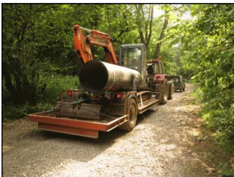
Photo 4. Excavator and pipe being transported to site, July 2013. [Photo: Graham Price]
