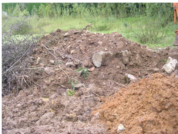
Photo 2—Infill from holes 2 and 3
