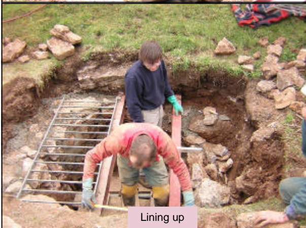
Lowering the RSJs into position
